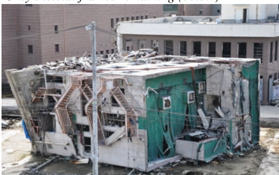
Onagawa town, overturned building (above) Only skeletal frames remaining (below)
